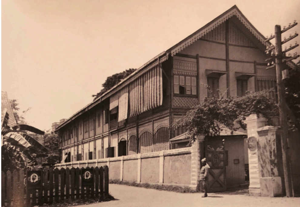
Figure 4-49: Back of the Chancery Building viewed from Soi Rongparasi Source: La Residence De France A Bangkok , 2015, 97
