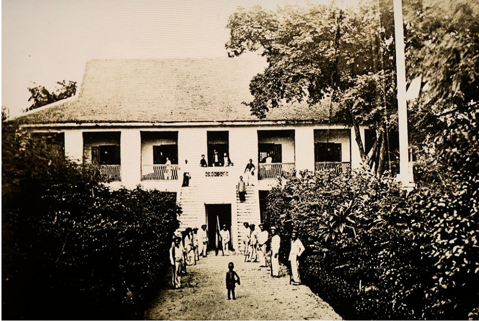
Figure 4-50: The French Consulate in Bangkok, 1866. Source: La Residence De France A Bangkok, 62-3
