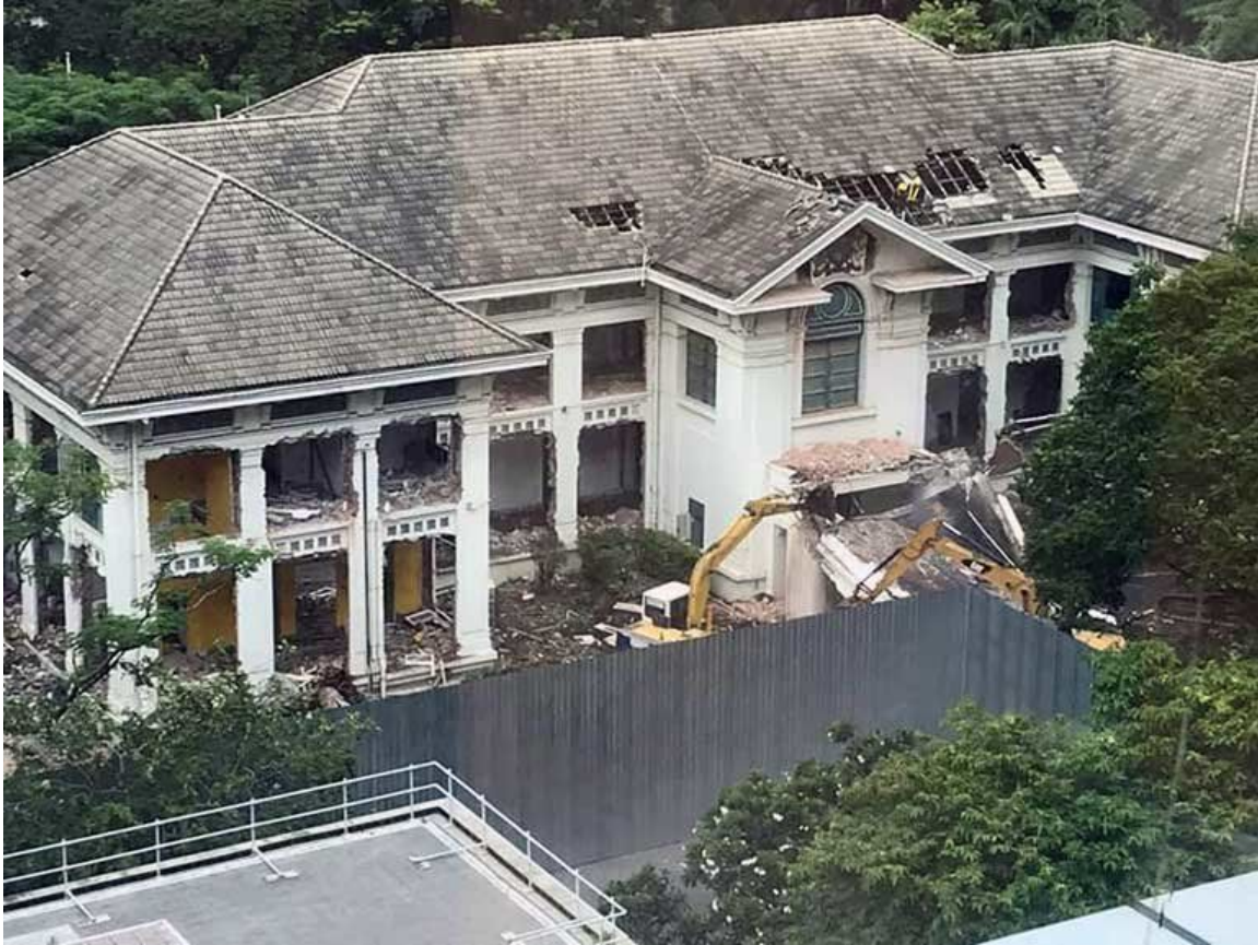
Figure 4-23: The demolition of the British Embassy, 2019
