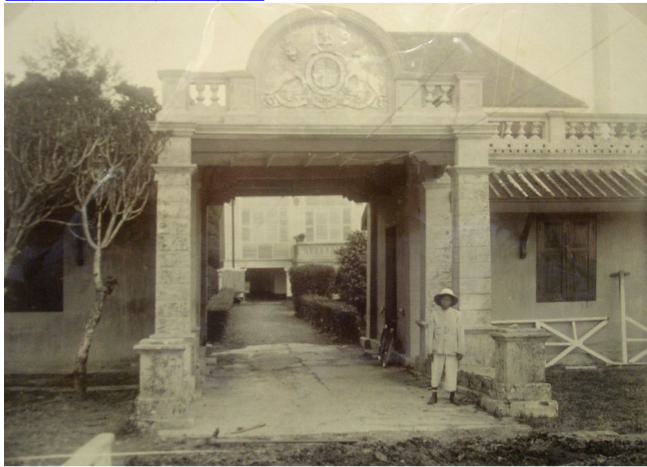
Figure 4-15: The gate lodge located between jetty and the residence, 1907.
