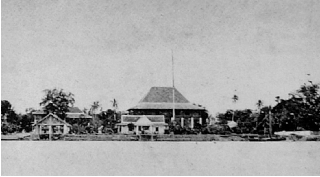
Figure 4-6: British Consulate complex, which had a flagstaff and a gate lodge in front of the residence, viewed from the river, 1867
